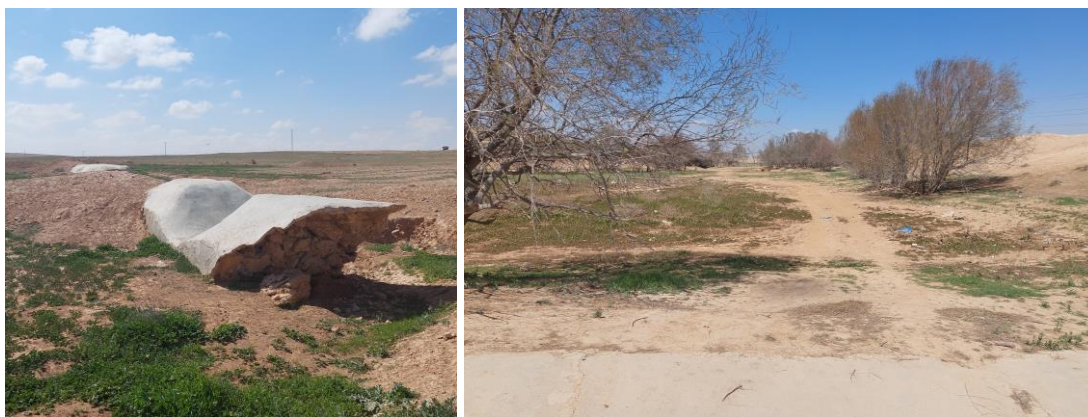
Figure 1. Broken flood water spreading structure (left), and one of the dam reservoirs completely filled with sediments (right).
